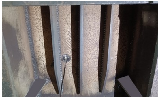
Figure 4. Picture of the sensors installed on the side shell.
