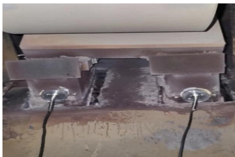
Figure 6. Picture of the sensors installed on the collector bars.
